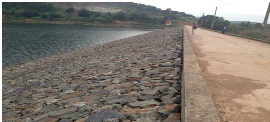
Figure 3: Current status of the Dong Do upstream dam roof
