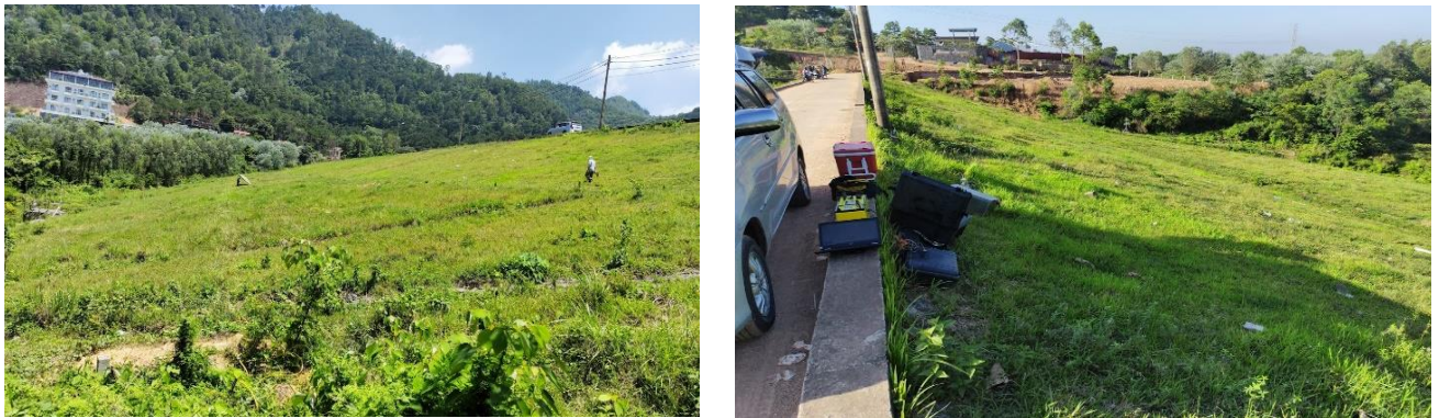
Figure 2. Current status of the Dong Do downstream dam roof
